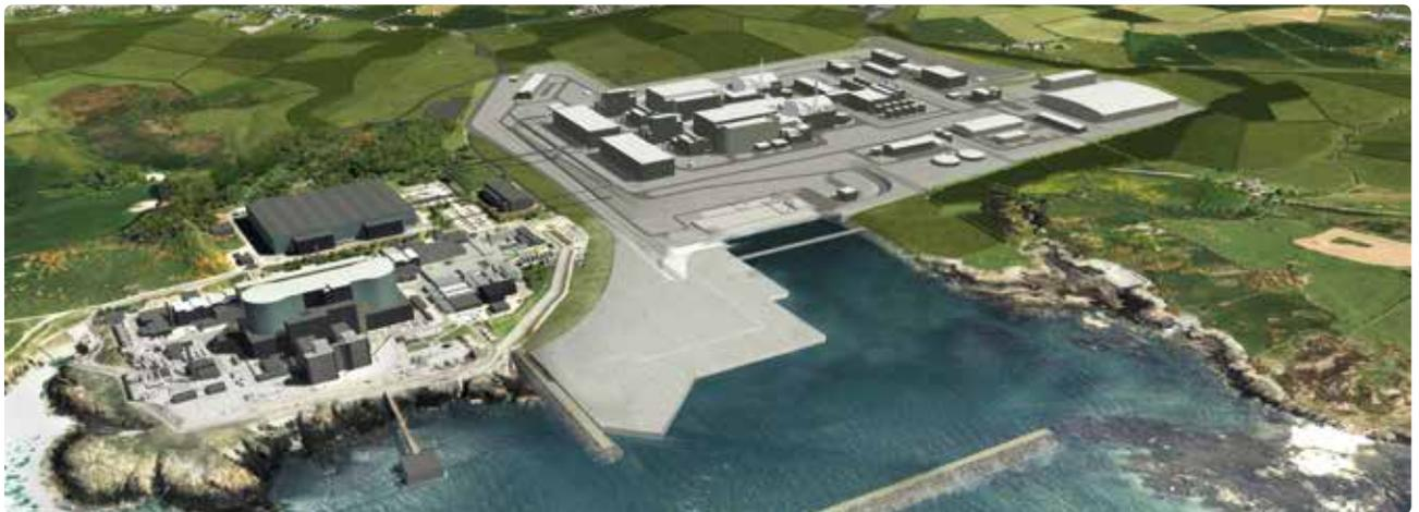
To construct the Wylfa Newydd Power Station, we are proposing to bring between 60% and 80% of our bulk materials to site by sea. We will do this at a specially constructed Marine Off-Loading Facility (MOLF) at Porth-y-Pistyll.
